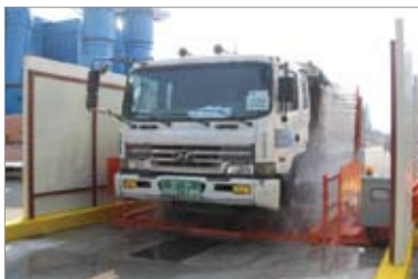
Vehicle Wheel-Washing Facility in Operation
